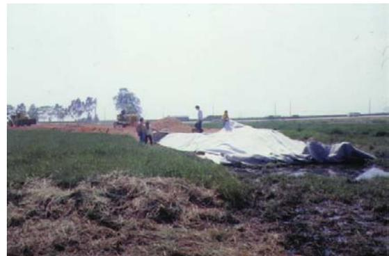
Construction of a reinforced unpaved road on soft organic clay
