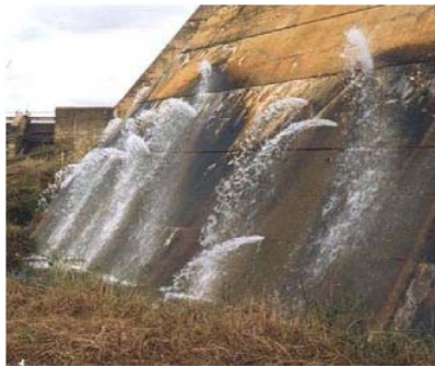
Leaking dam (*)
