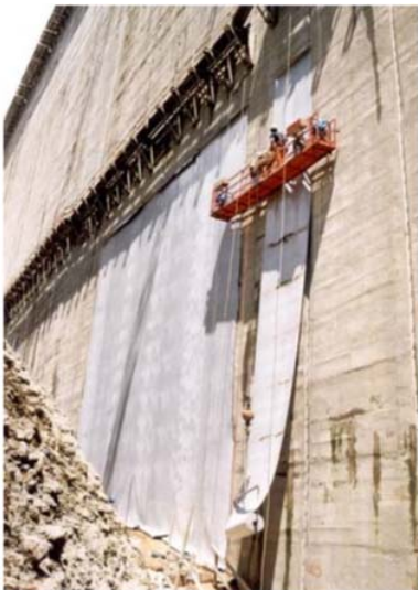
Lining the upstream face of a dam (*)
