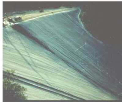
Geomembrane-lined dam (*)
